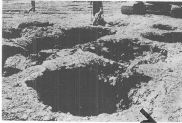
Figure 23. Ground heave induced by dynamic compaction.
